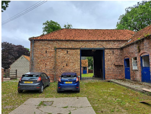
View of main barn indicating slot openings and large door openings to west (and east) elevations
