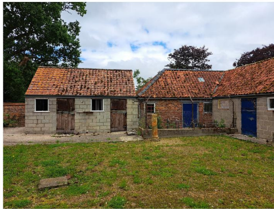
View of modern blockwork intervention
