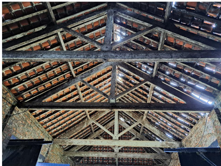
View of trusses to main barn
