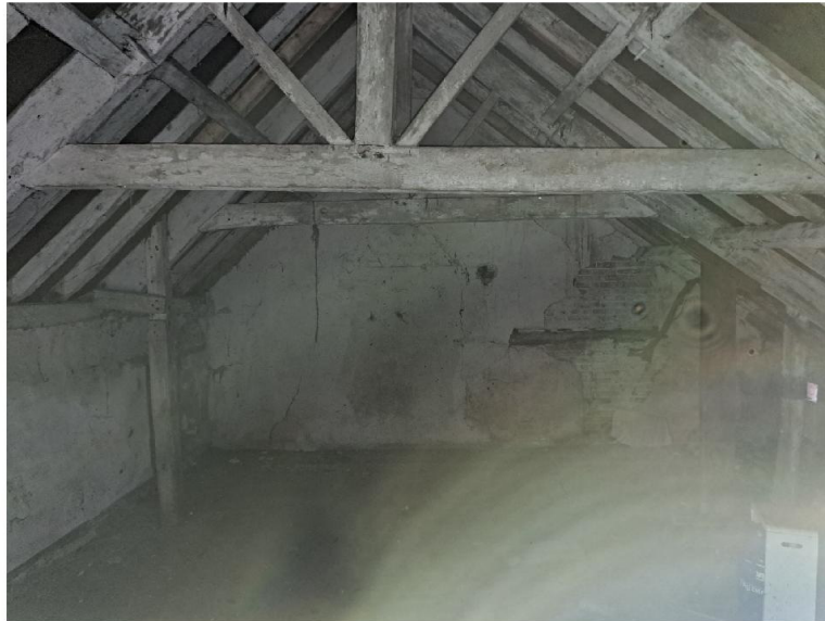
View of trusses at First Floor
