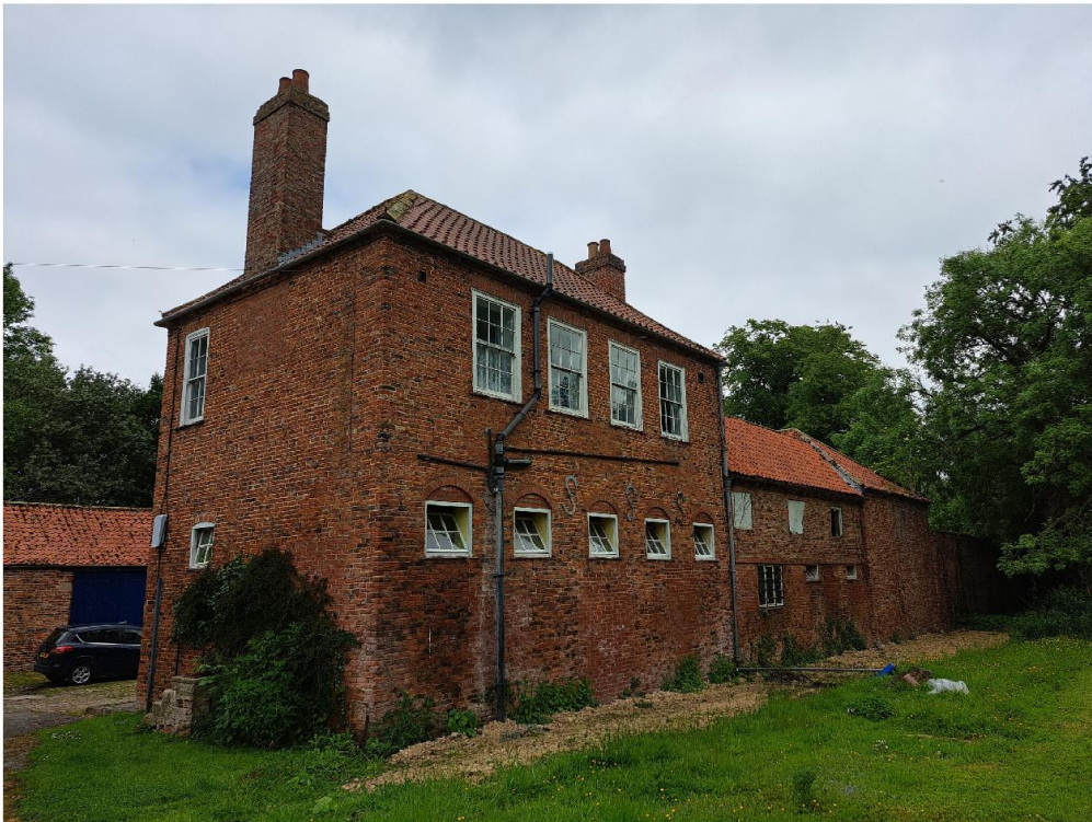
VIEW OF EXISTING BUILDING
